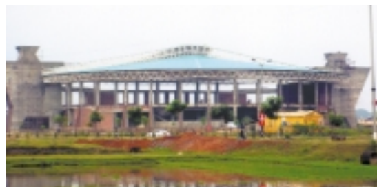
Austnam roof on new swimming stadium for South-East Asia Games, Hanoi.
