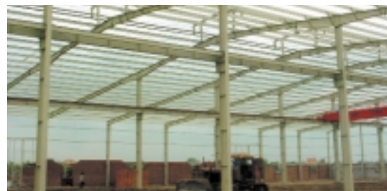
An Austnam factory building under construction.
